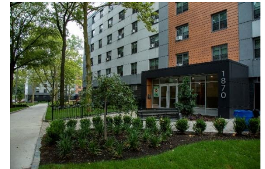
Site improvements at Baychester
